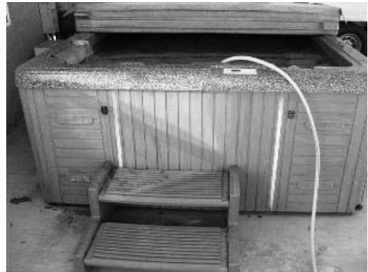
Figure 8.1a Indirect Cross-connection
