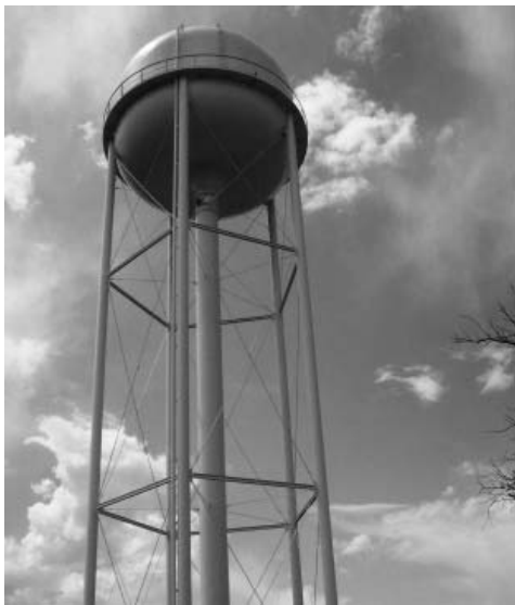
Figure 7.1.5a. Elevated Steel Tank
