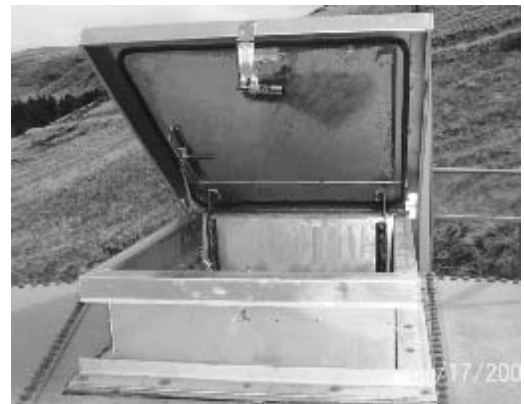
Figure 7.1.5b. Shoebox Lid on Tank Access
